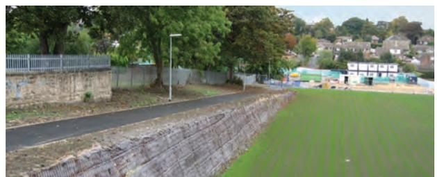
*With construction successfully completed, the TensarTech GreenSlope can be prepared for the vegetation stage.*
