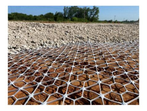
Highest performing geogrid for soil stabilization that combines advanced material science and optimized geometry to solve civil and site construction challenges.
