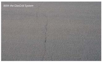
Pavement surface condition following 11 years of post-rehabilitation service.
