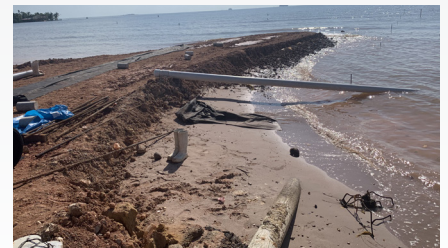
Very soft sandy silt with low bearing capacity, posed significant challenges for stability.
