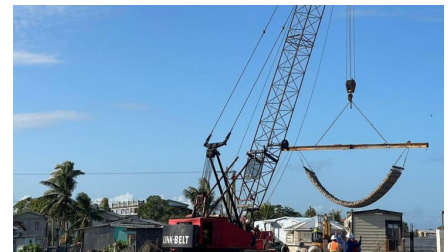
Despite having no prior experience, the contractor pre-fabricated the TRITON® mattresses and completed installation using standard construction equipment and crew.
