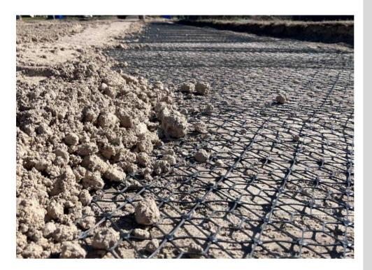
High performing geogrid with optimized geometry providing solutions for civil and site construction challenges.
