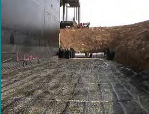
To eliminate costly concrete foundation walls with drilled shaft foundations, the John Paul Jones Arena at the University of Virginia combined the SierraScape® System Pressure Relief Wall with the Tensar Geopier System for foundation improvement.
