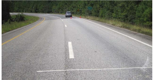
The GlasGrid reinforced section was also evaluated in 2018. After 60 million ESALs, cracking was starting to appear but limited to the 18 yr. old construction joint.
