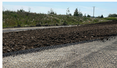
H-series geogrid offered a higher performing solution compared to the original TX5 geogrid specification.
