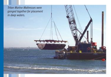
The project crew used a four-point lifting frame and a combination of shore- and barge-mounted cranes to lift and place each unit. Because of murky conditions on the underwater sections, the lift operator used sighting aids to facilitate mattress placement.
