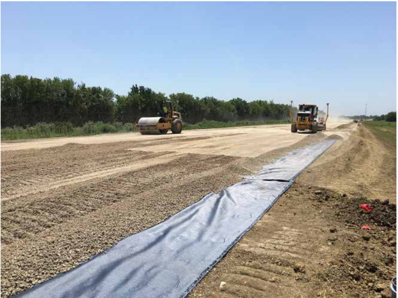
Figure 3. Roadway construction over geotextile.
