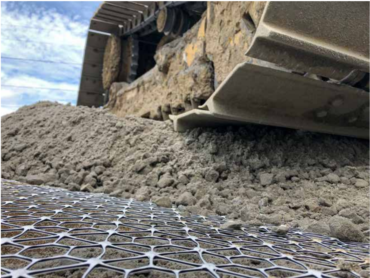
Figure 4. Soil placement and compaction over geogrid.
