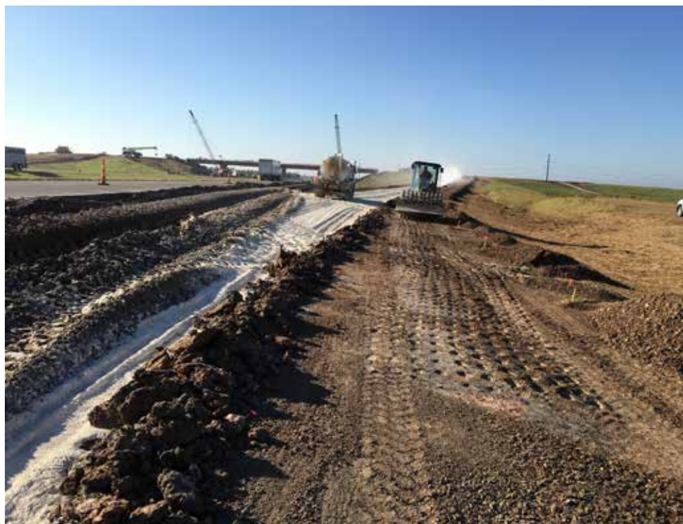
Figure 2. Regrading and compaction of lime-treated subgrade soil.
