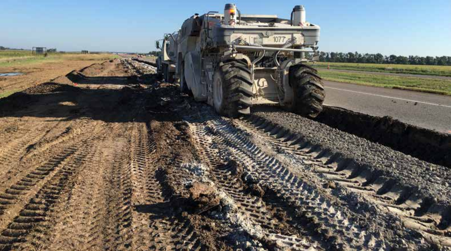
Figure 1. Lime application and mixing during roadway subgrade stabilization.
