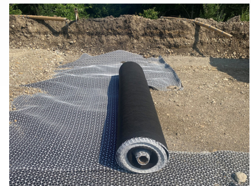
InterAx FilterGrid and InterAx NX850 along with existing materials were used to create the mechanically stabilized layer.
