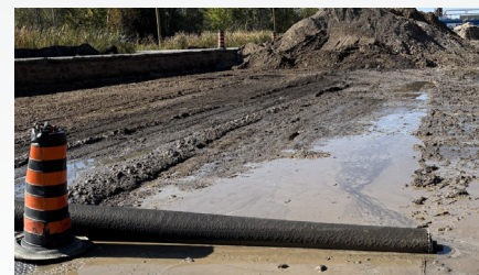
Low CBR values made conventional construction methods impractical.
