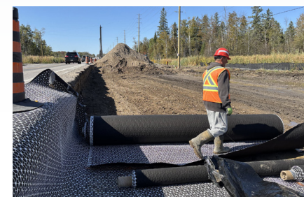
Tensar geogrid technology allowed construction to proceed over challenging peat deposits.
