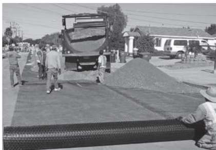
Geogrid should overlap in the direction of advancing fill.
