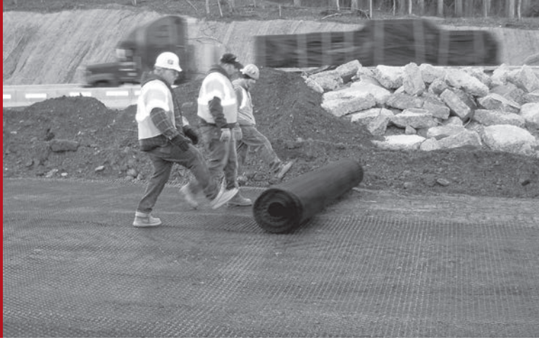
Rolling out Tensar® Geogrid.
