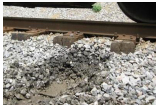
Even where track was observed to have dropped there was no movement evident under traffic.
