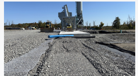
The InterAx® design delivered long-term durability without unnecessary construction expense.
