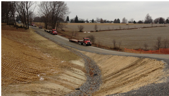
TriAx Geogrid proved to be extremely effective in stabilizing soft soils for the Rex Energy well pads and access roads.
