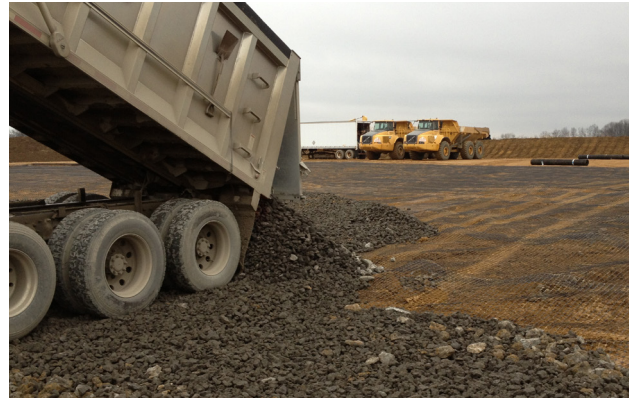
Tensar® TriAx® Geogrid was installed at the Warner and Bame well pad sites to stabilize soft soils.
