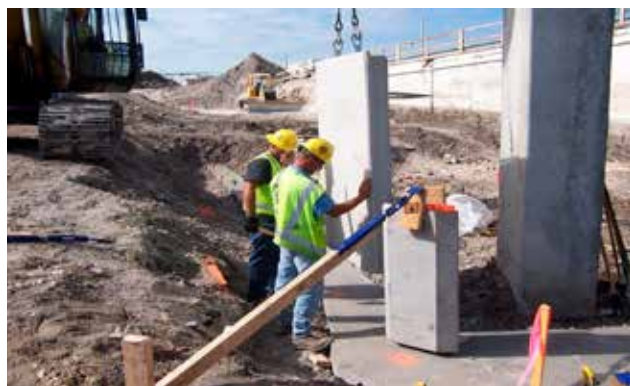
IMAGE G: Placement and bracing of concrete panels.
