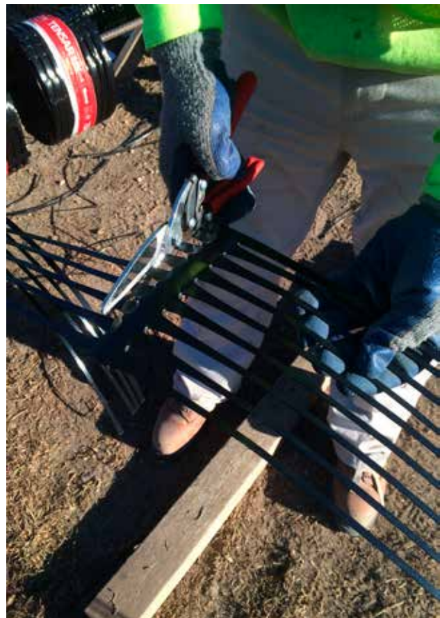
IMAGE E: Safe cutting of Tensar Geo-Strip can be done with a variety of cutting tools. Care should be taken to avoid cutting the transverse bar.
