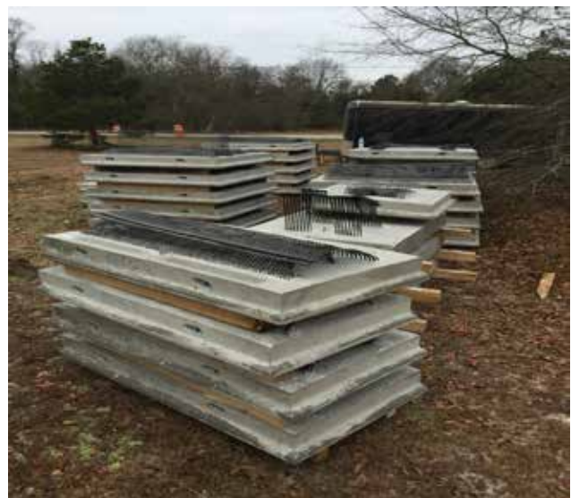
IMAGE B: ARES panels should be stacked on a level, stable surface provided by the Contractor. Dunnage shall be carefully selected to allow panel separation and placed to avoid panel cracking.
