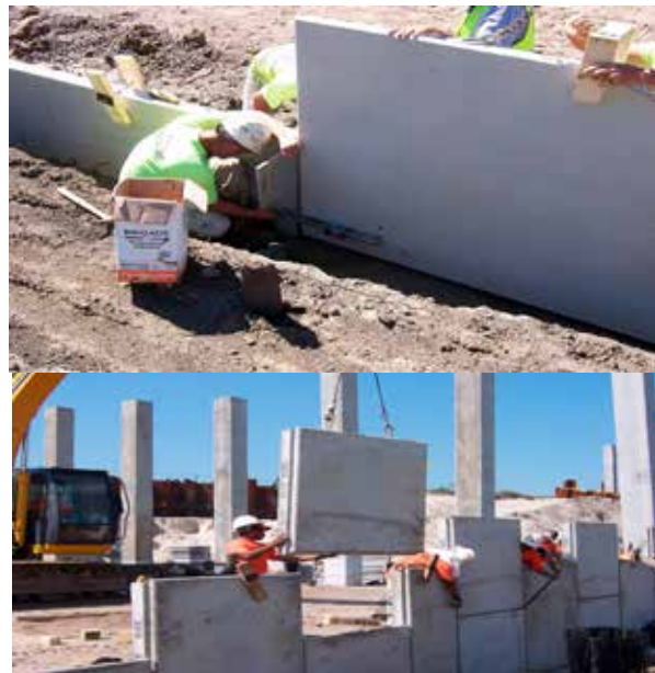
IMAGE I Placement of 5 x 5 panels. Subsequent course: panels placed, positioned, aligned, clamped, battered and wedged. All but the top course are backfilled.
