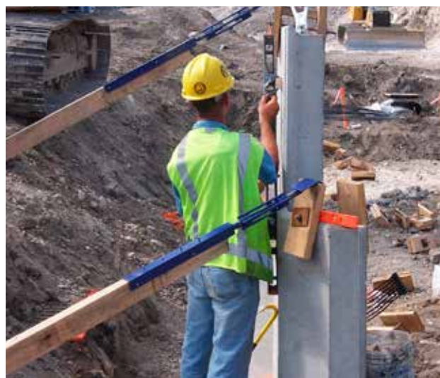
IMAGE H: Establishing batter of ARES® panels.
