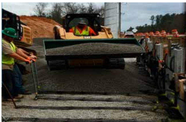
IMAGE 0: Placement of fill on tensioned Tensar Geo-Strip.
