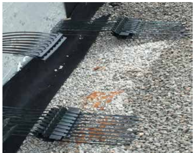
IMAGE K: Area immediately behind panel may be left open until Tensar Geo-Strip is covered by one lift of compacted backfill.
