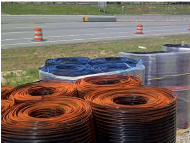
IMAGE C: Color coding of geogrid panels allows for quick, accurate identification even after labels are removed.
