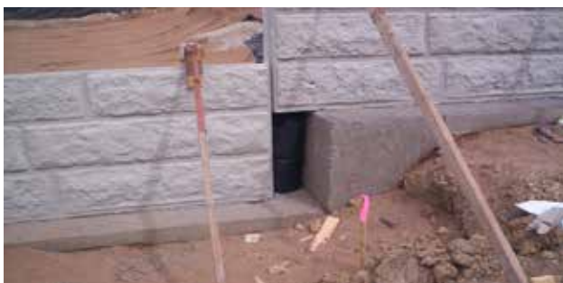
IMAGE E: Upper leveling pad offset 9 in.
