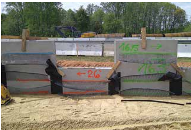
IMAGE D: Color-code the geogrid tabs on each panel to correspond with the geogrid rolls.
