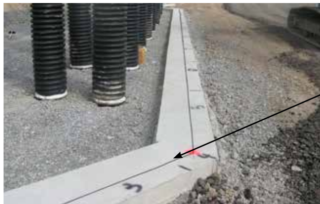
IMAGE F: Recommended location of chalk line on leveling pad.
