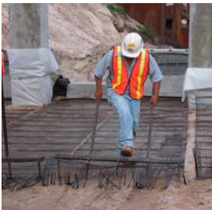
IMAGE L: Tensioning of uniaxial geogrid or single layer Tensor Geo-Strip prior to fill placement.
