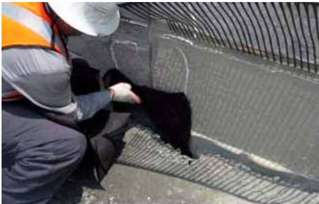
IMAGE J: Placement of filter fabric at ARES® vertical joint.
