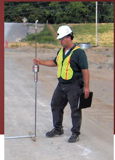
Analyzing local soil conditions
