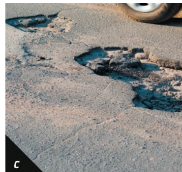
Inadequate pavement structure as depicted by A ) alligator cracking, B ) block cracking and C ) spalling due to excess moisture within the structure.
