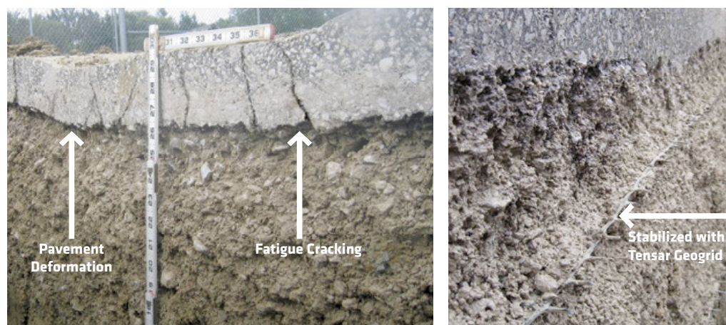
FIGURE 10 The post-trafficked trench section (right) reveals a dramatic reduction in asphalt and aggregate deformation due to the inclusion of Tensor Geogrid when compared to the unstabilized section (left).
