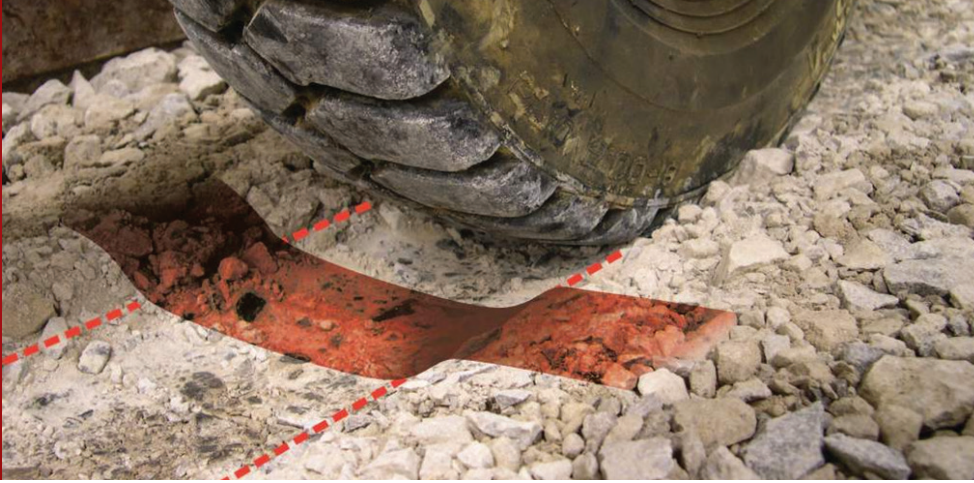
Rutting accumulation at the surface and the subgrade were used to compare geogrid performance.
