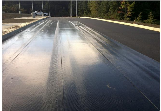
*GlasGrid TF with pre-installed tack film was installed in the bus and traffic areas to reinforce the pavement.*
