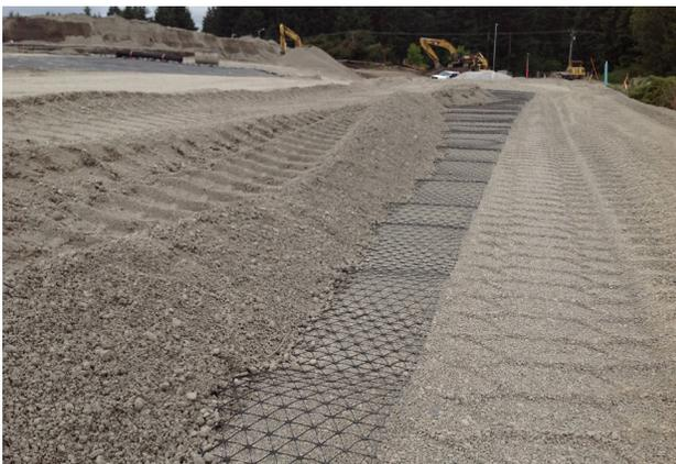
*Tensor® TriAx® Geogrid was installed to help resolve soil stabilization challenges over the capped landfill.*
