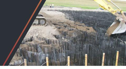
When faced with soft foundation soils where expensive piling and other deep ground improvement solutions are not viable or too costly, the Tensar Stratum™ Cellular Foundation Mattress System provides an alternative approach for construction, often delivering savings in cost and time.
