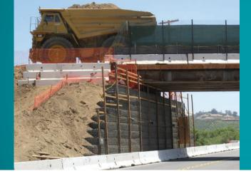
The photo to the left illustrates a CAT 777 weighing approximately 360,000 lbs that is supported by a Tensar Temporary Wall as it drives to the embankment site.
