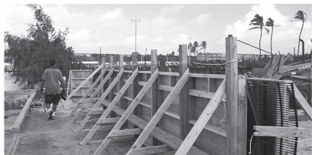
IMAGE 3: This wooden filling frame was constructed for a marine mattress project in Kauai, Hawaii.
