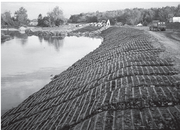
IMAGE 6: Completed installation for riverbank protection.
