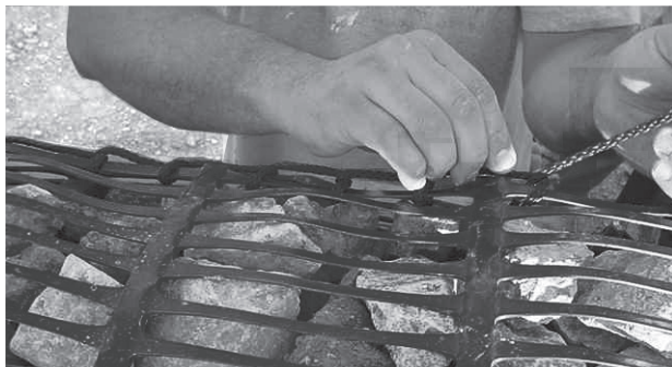
IMAGE 1: Knots should be tied in a manner to prevent slipping and cinching.
