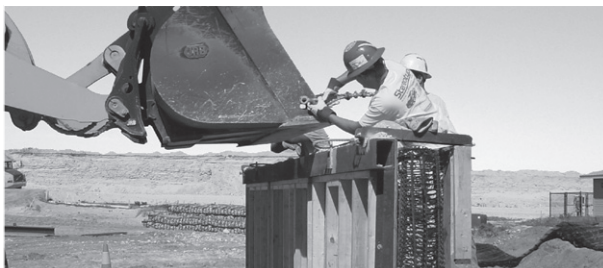
IMAGE 4: Overfill so that stone is heaped slightly above the top of the unit.
