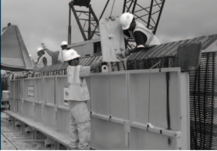
Plywood spacers help hold the two main layers of grid apart, helping to fully open the mattress for filling.
