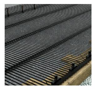
Once the connectors and the geogrid are in place, the Olympia<sup>®</sup> Units must be swept clean prior to placing the next course. Failure to do this can result in problems with seating and leveling of subsequent courses.
