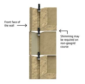
If the design dictates the need for a geogrid at a particular elevation, install the Tensar<sup>®</sup> Geogrid with the teeth of the Olympia Connectors penetrating through the geogrid apertures. The pin should never be utilized to connect the geogrid to the facing units.
