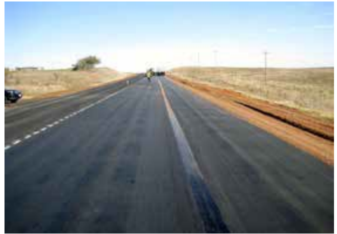
Image 3: All adjacent GlasPave should be overlapped.
