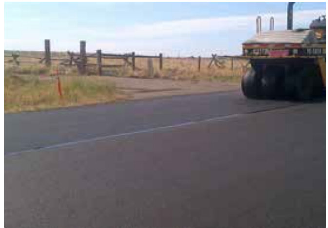
Image 4: Use a pneumatic tire roller to bond the GlasPave to the tack coat.
