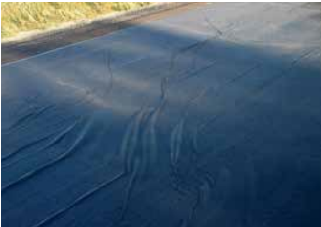
Image 5: Wrinkles after rolling that are 1 in. or greater should be slit and shingled in the direction of paving.
