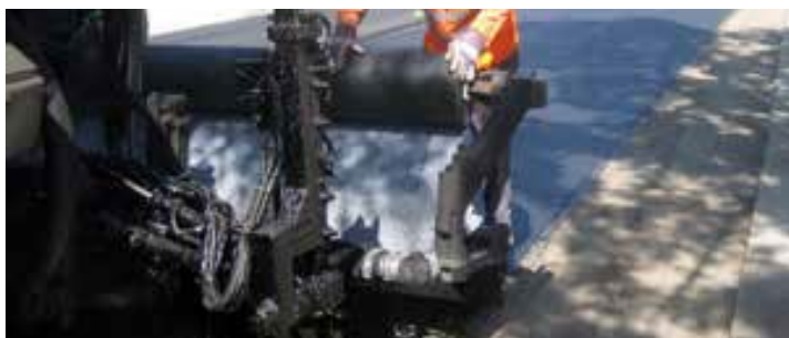
Image 2: Distributor truck with fabric applicator attached to the back.
