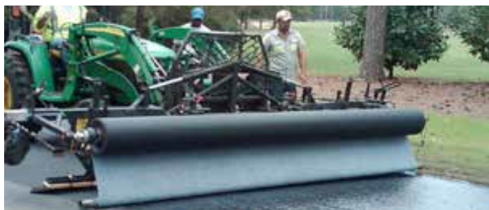
Image 1: Interlayer laydown equipment.
