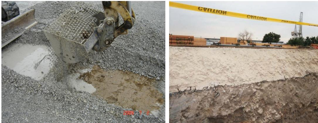
Figure 3 – Examples of trenching through sections with Tensar geogrids.
