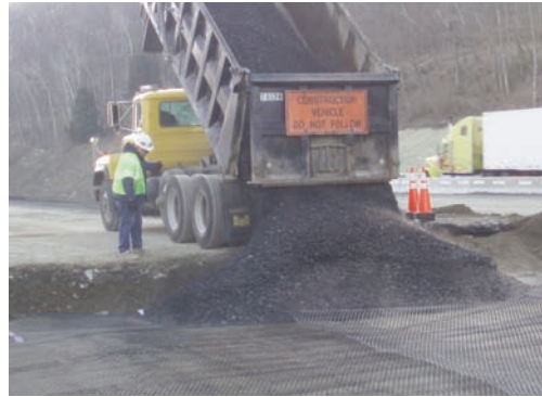
The Spectra® System using TriAx Geogrid provided a stable platform over weak soils.
