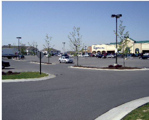
Tensar BX Geogrids helped these pavements handle both light and heavy-duty traffic.
