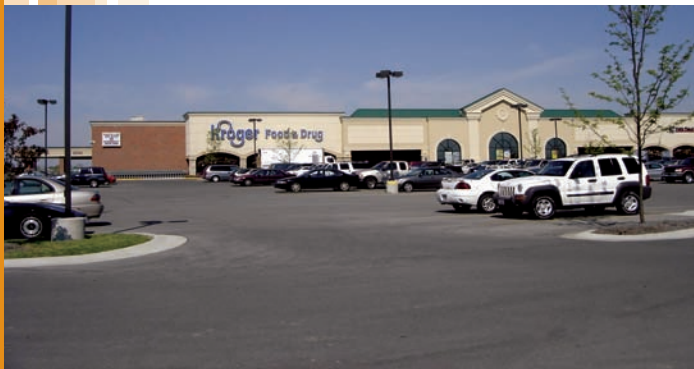
Tensar BX Geogrids offered a dual approach to cost savings for this Cincinnati area Kroger.
