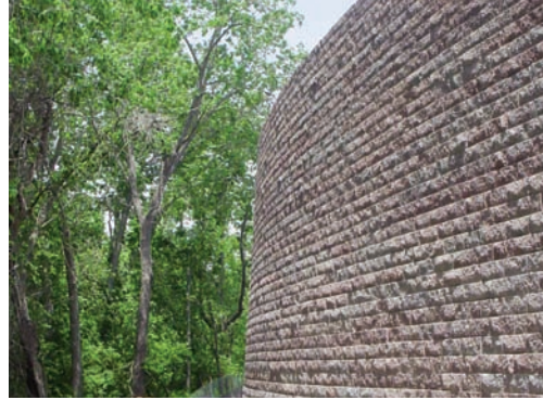
The Mesa System provided a structurally sound and attractive solution.
