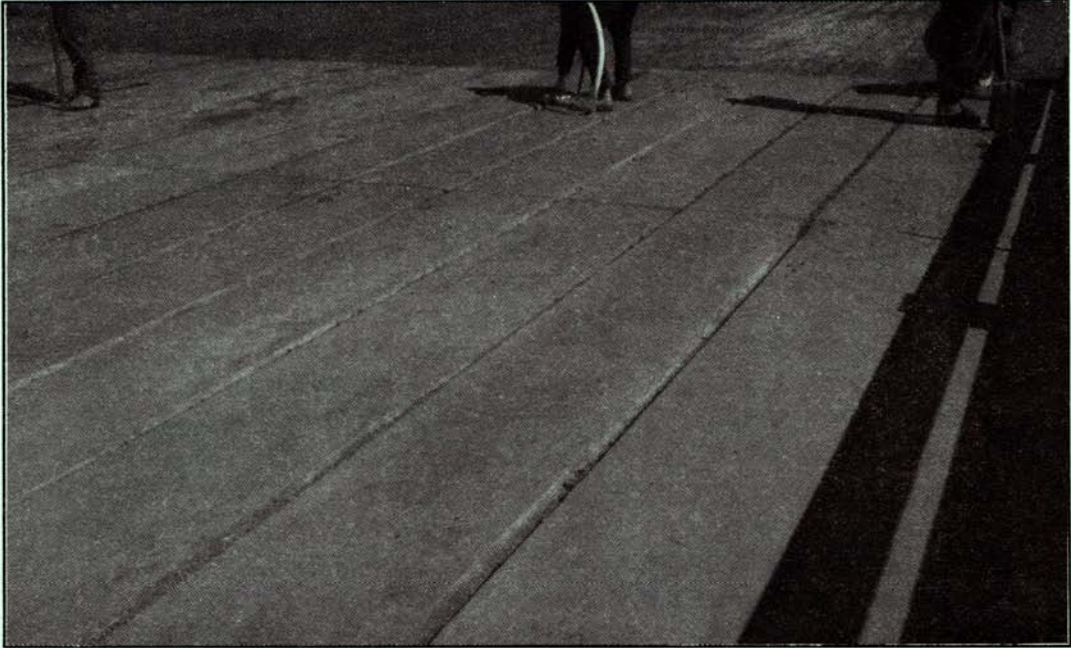
Mount Zero bridge U-form Beams.
