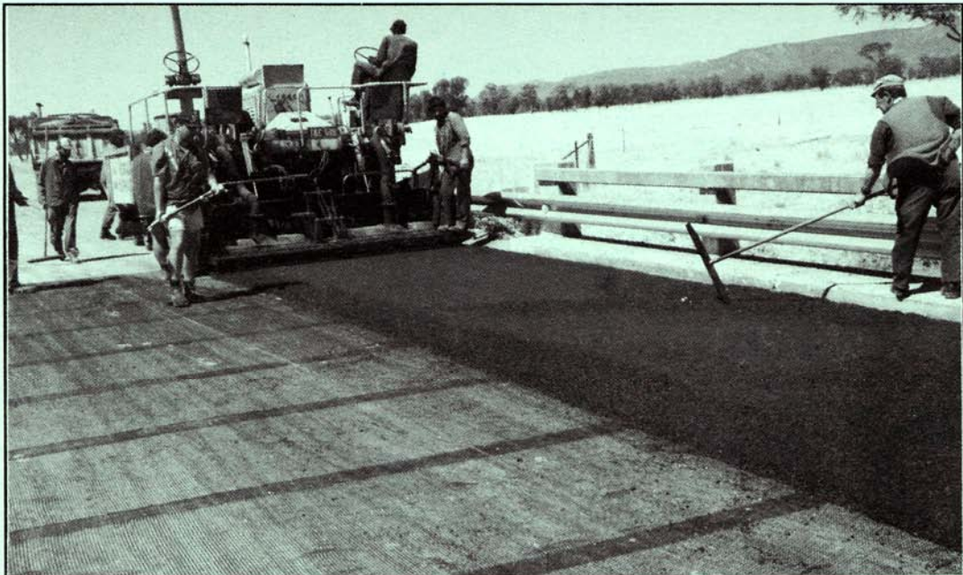
Placement of Intermediate course over GlasGrid*
