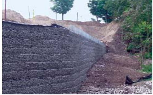
Construction of the 13.5 meters (44 feet) tall stone-faced wall started in June 2004.
