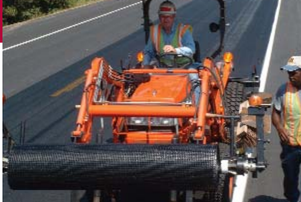
The grid is rolled out over a thin leveling course placed before the main asphalt overlay.
