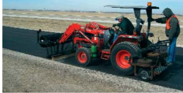
One step installation – The tractor unrolls the grid, and places it, while the roller on the back activates the adhesive on the grid.
