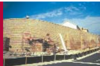
The finished wall bordering the property measured approximately 600 feet in length and up to 30 feet in height.
