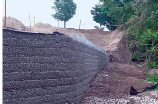
Construction of the 13.5 meters (44 feet) tall stone-faced wall started in June 2004.
