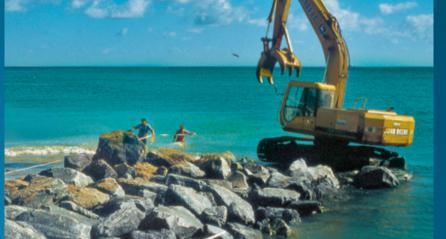
Tensar® Geogrid composite eliminated the need for steel sheet piling for sand tightening this structure.
