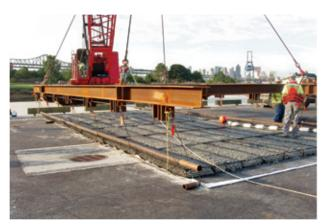
Triton® Marine Mattresses have been deployed as part of a reactive capping system for the remediation of NAPL when used with CETCO® Reactive Core Mats.®
