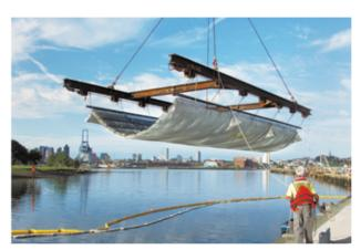
Triton Marine Mattresses have been used to provide effective capping for a wide range of contaminated sediment projects.
