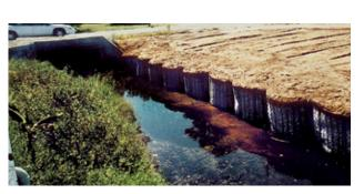
Triton Circular Marine Cells anchored by Tensar® Geogrid, provide economical, easy-to-install solutions for applications like this channel wall in a residential community.
