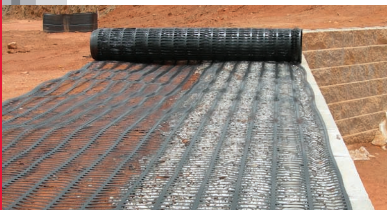
LH800 Geogrid is rolled out parallel with the wall or slope face for easy installation.
